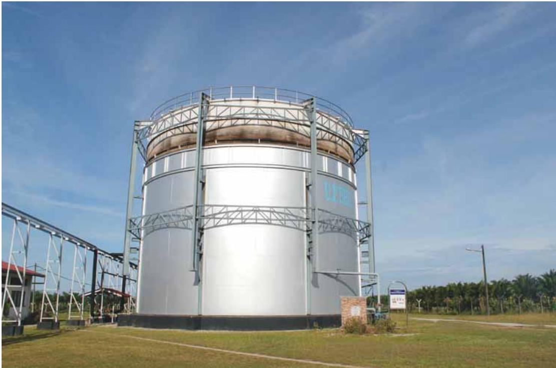
*The Jendarata Estate Biogas Plant commissioned in 2006 treating the Palm Oil Mill Effluent. In the process of reducing the Biochemical Oxygen Demand by 99%, biogas is produced by methane bacteria and subsequently used as a source of green energy.*
