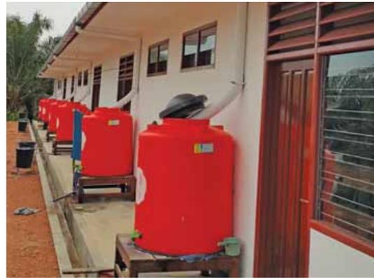
Water tanks are supplied for harvesting rain water.
