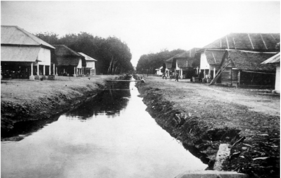
Jendarata estate workers' housing, 1919
