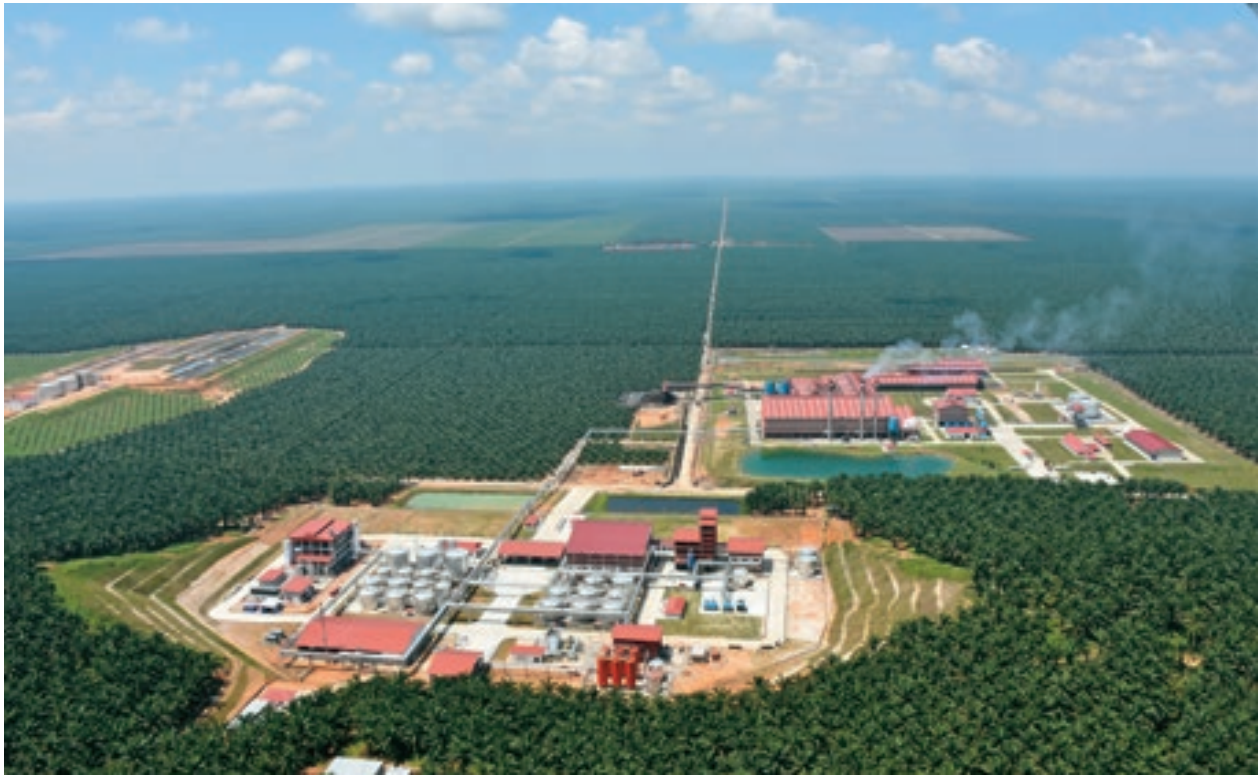
The Optimill and Unifuji project encompassing an example of the “circular economy”. An enormous effort was undertaken by many to complete this state of the art project.
