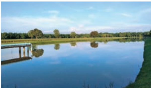
The water reservoir at Jendarata Estate.
