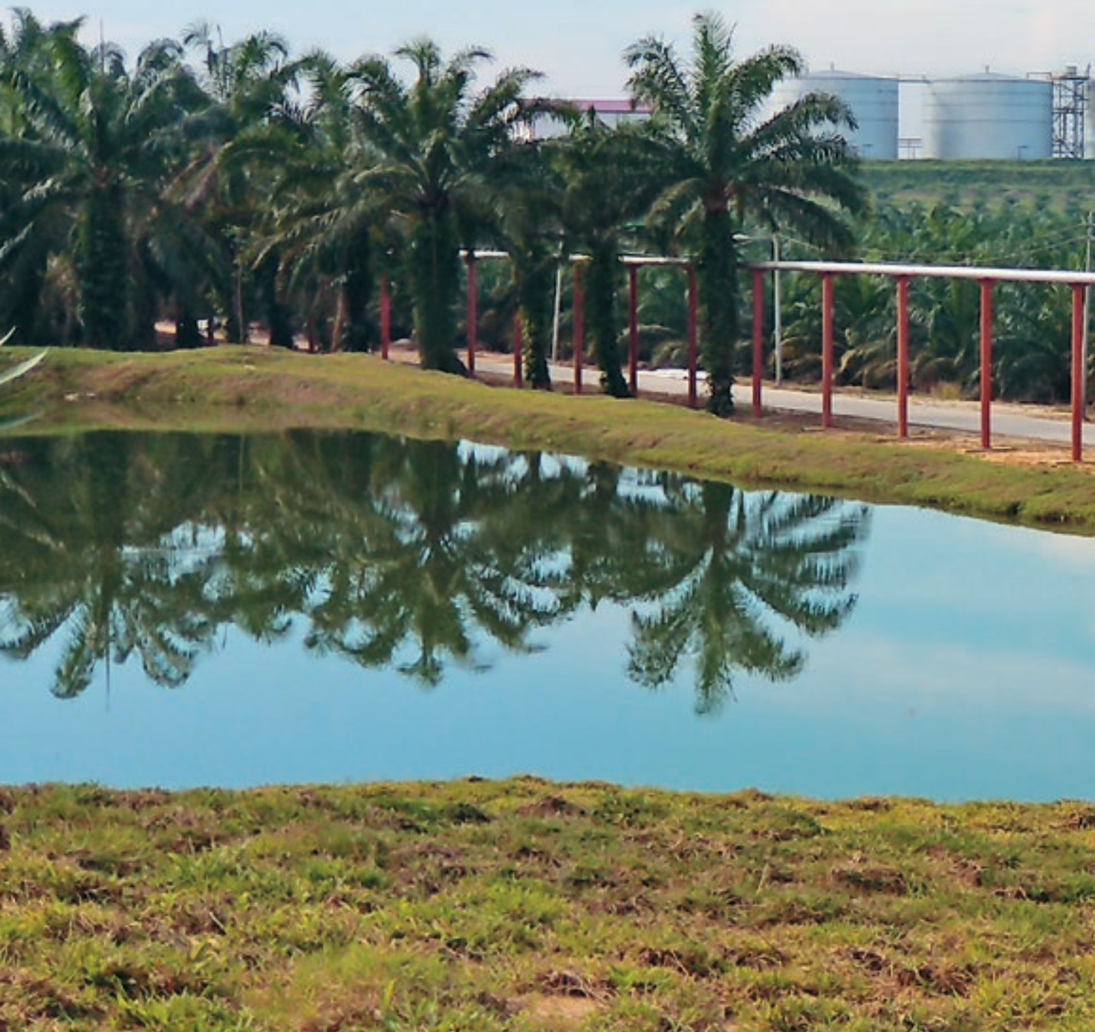
The latest and largest Biogas Plant built in 2017/2018 located at the Optimill and generating electricity which is used internally.
