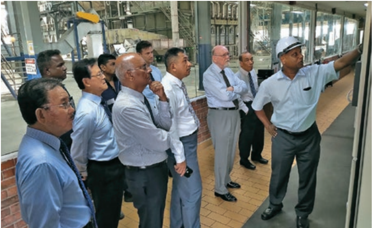
Mr. P. Seker, Director of Engineering, Upstream giving a briefing to the members of the Board in the Power Control Room at the Optimill.
