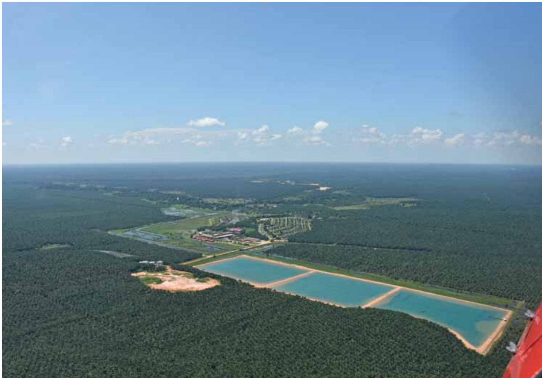
The Ulu Basir water reservoir established to cater for the Optimill water requirements.
