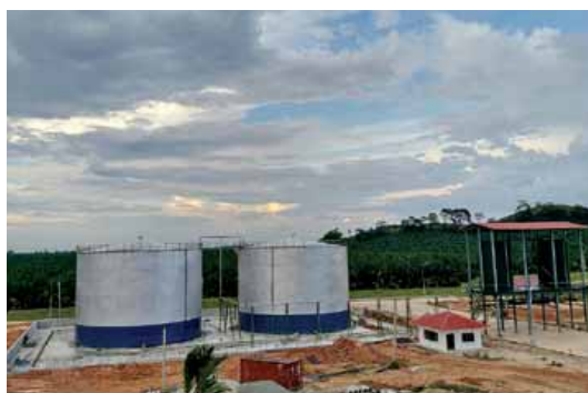
CPO storage tanks.
