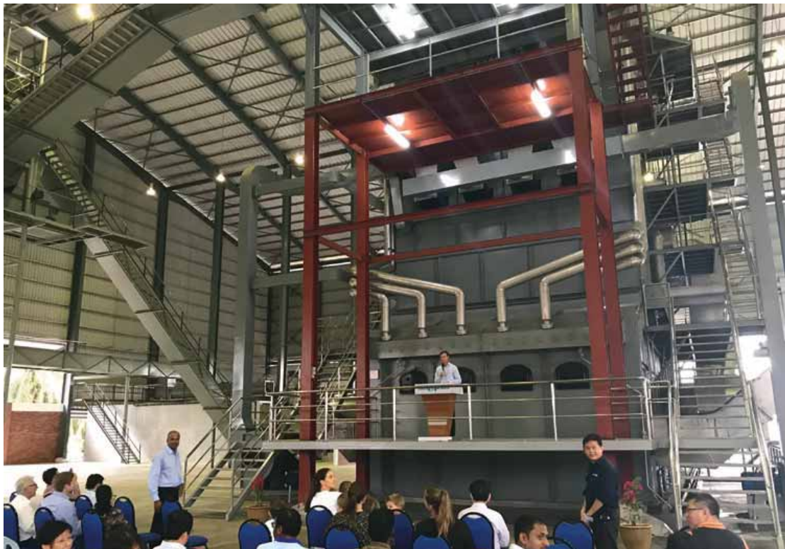
Official opening of the Jendarata Biomass boiler No 2 at Jendarata Palm Oil Mill in December 2017.
