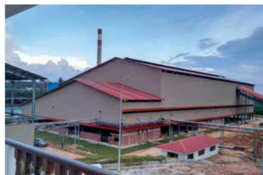
The new Biomass Boiler power plant.
