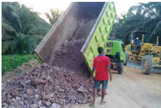
Roadwork repairs towards PT Medco to assist local communities.
