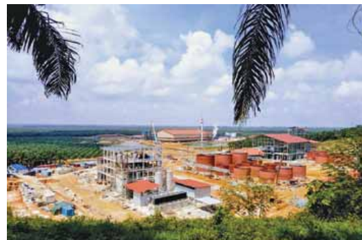
UniFuji refinery construction site with the Optimill in the background.
