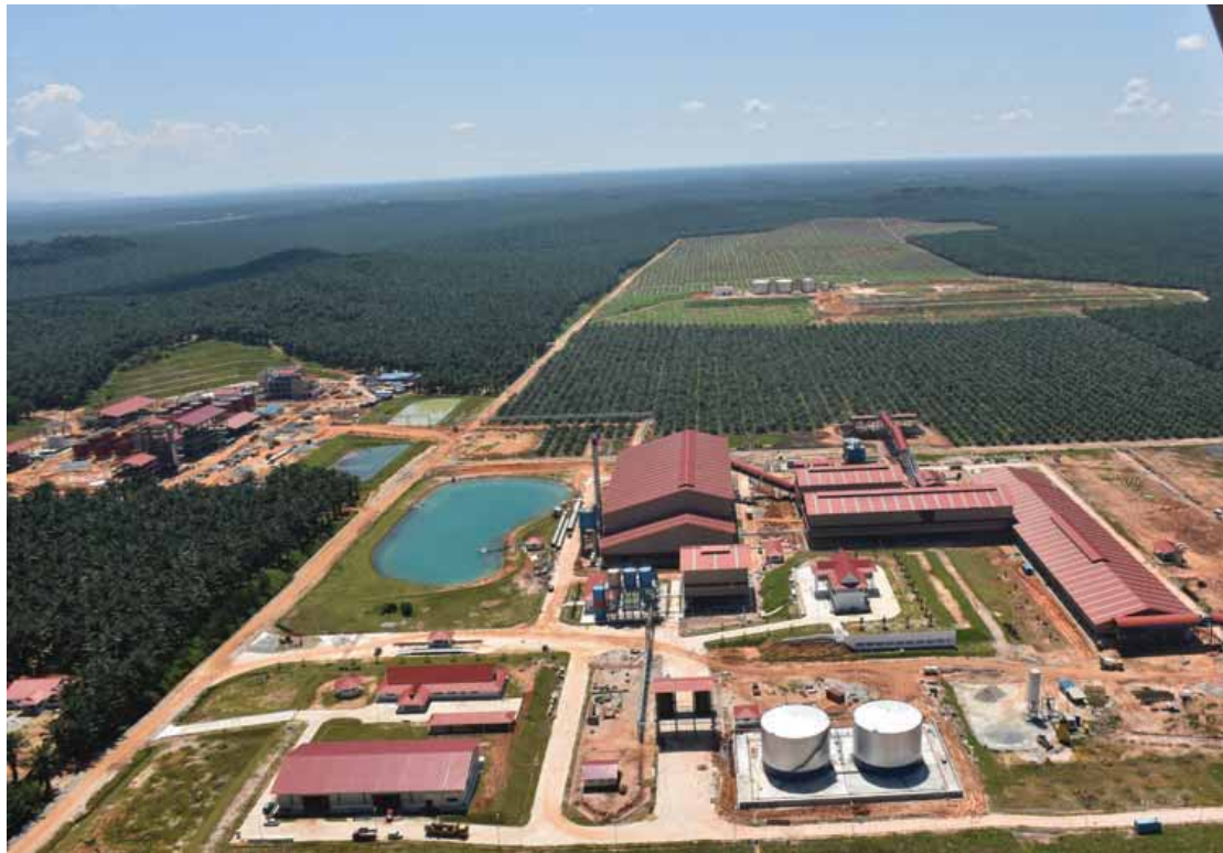
The state of the art 60tph Optimill site located at Ulu Bernam on the very grounds where United Plantations undertook its large scale cultivation of oil palms in 1926. In the background one can see the modern biogas plant. To the left one can observe the UniFuji Refinery currently under construction.
