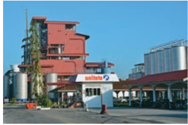
The Unitata inland refinery.
