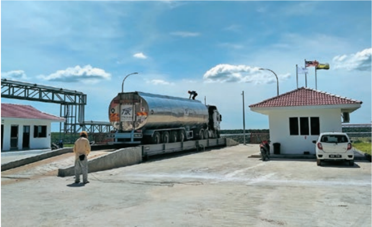
The weighbridge at the UniFuji Refinery.
