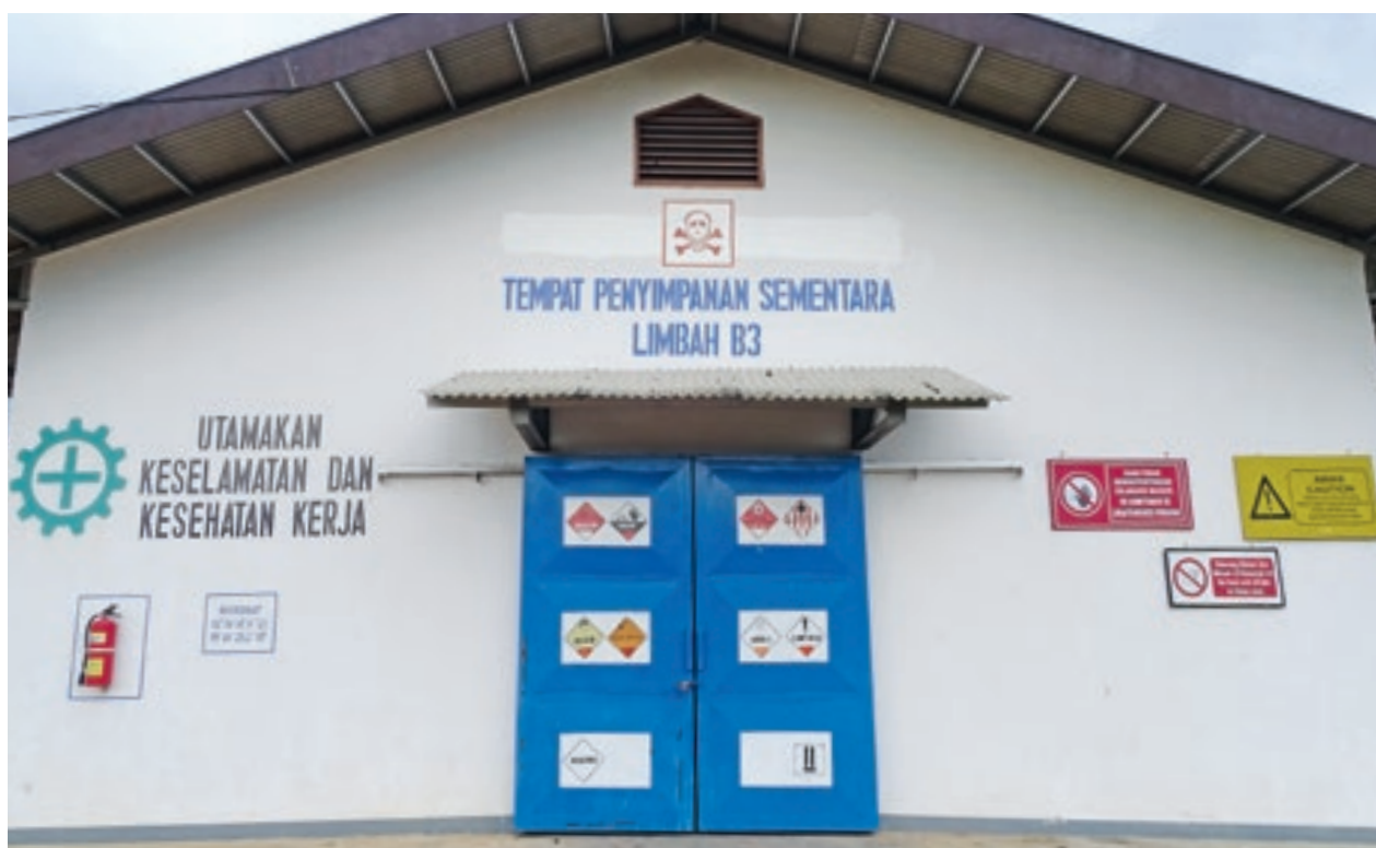
Temporary storage unit for used pesticides containers and schedule waste prior to recycling.
