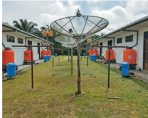
Water tanks are supplied for harvesting rain water.
