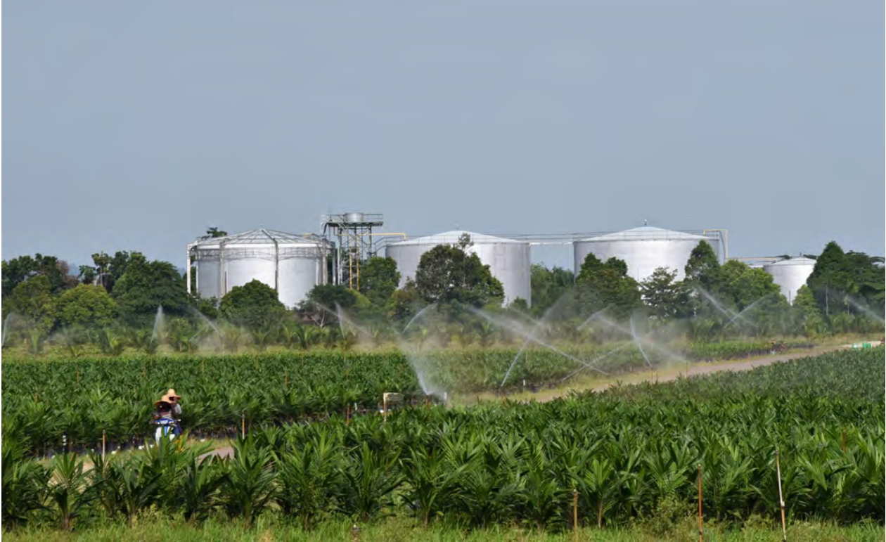
Biogas capturing facilities have been introduced on all our palm oil mills. Pictured here is the biogas plant at UIE.
