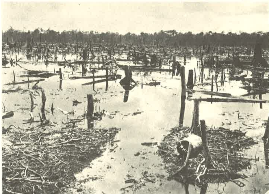
Flooding of low lying area at Ulu Bernam Estate 1930
