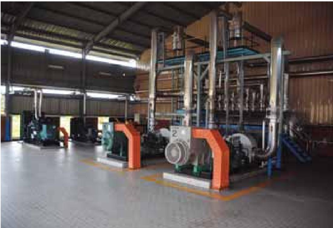
*The Engine Room displaying 2 x 1.4 mega watts turbines at the Lada Palm Oil Mill.*
