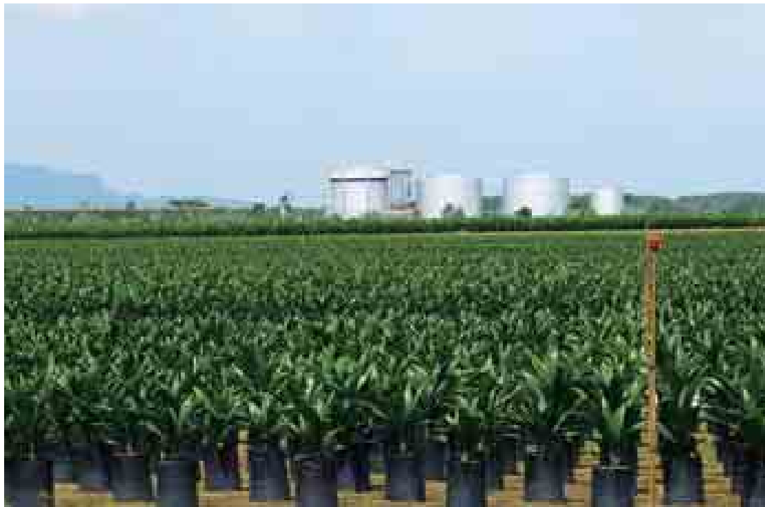
The biogas plant at UIE with the nursery at the forefront.
