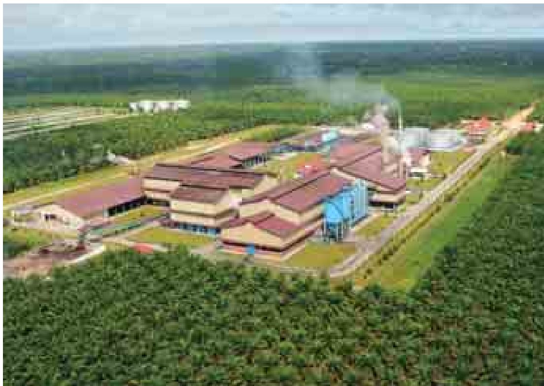
A modern Mill at Lada Estate with a biogas plant to reduce our Carbon Footprint.
