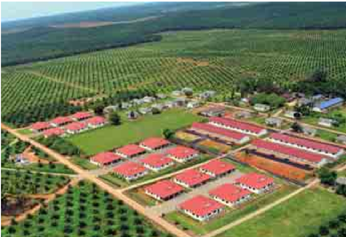
Modern housing both semi-detached and apartment blocks are completed at Lima Blas Estate.
