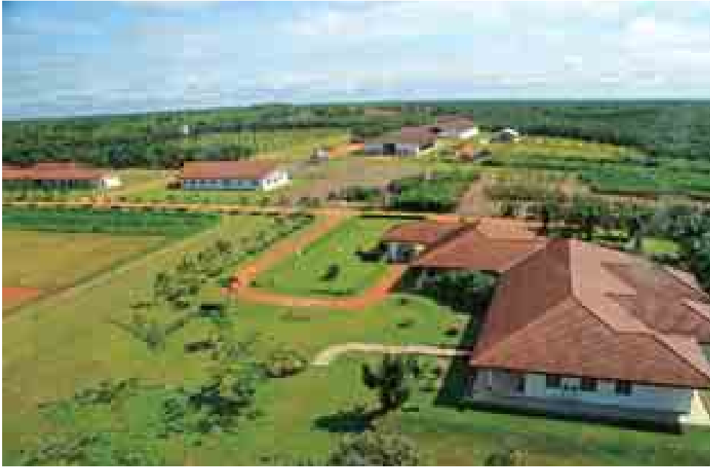
Modern Hospital/Health Care Centre at Lada Estate, Central Kalimantan.
