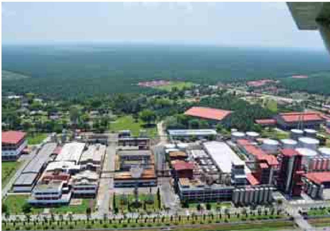
An aerial view of Unitata refinery.
