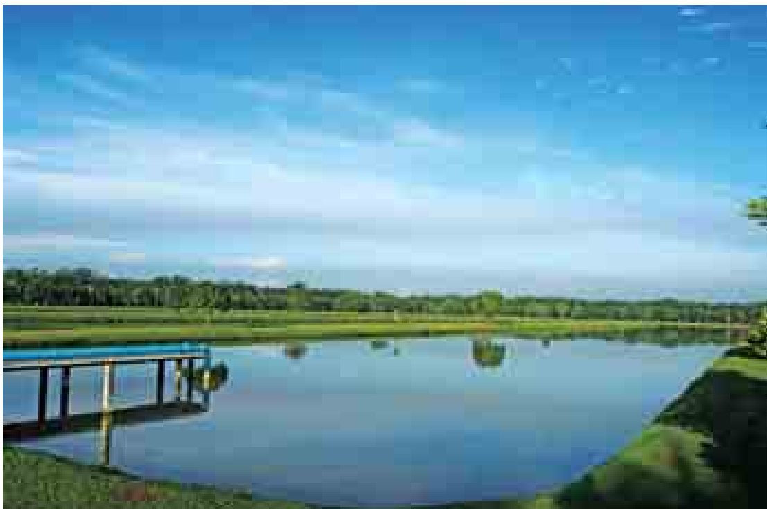
Reservoir at Jendarata securing clean and stable supply of water for the mill.
