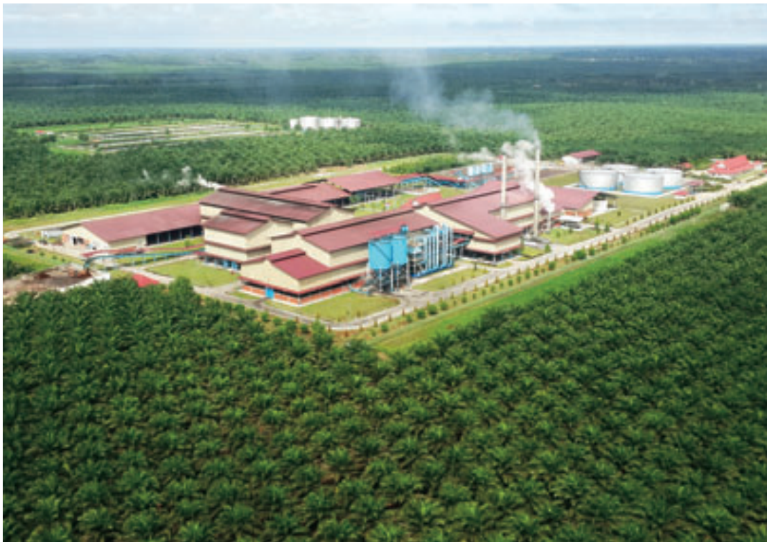
The Lada Palm Oil Mill is capable of processing 60 MT of fresh fruit bunches per hour. In the background one can note the Biogas plant.
