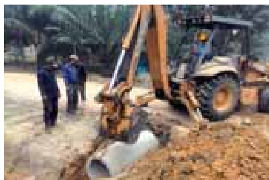
Repairs to road and culverts of adjacent villages at PT SSS
