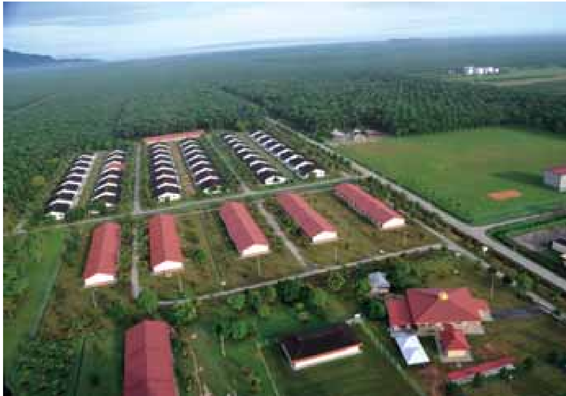
An aerial view of modern workers' housing complex at UIE estate in the midst of luscious growing oil palms.
