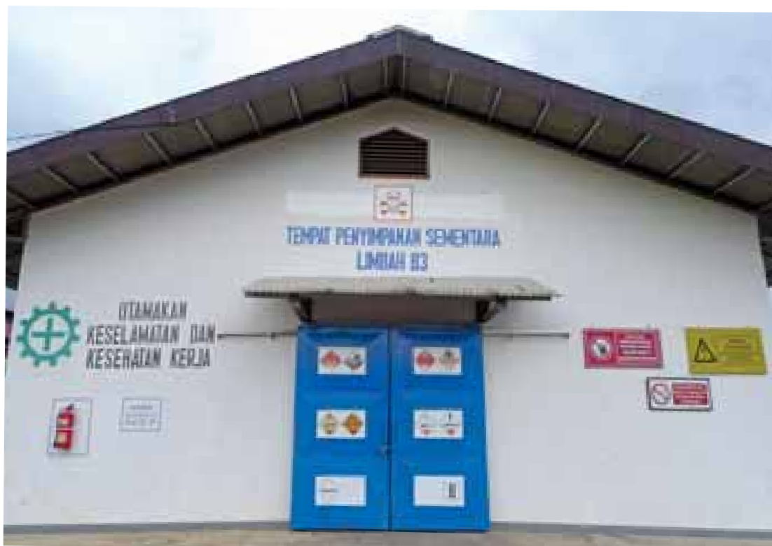
Temporary storage unit for used pesticide containers and schedule waste prior to recycling.
