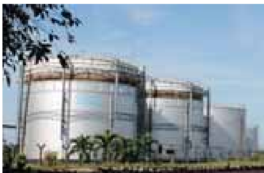
Our first Biogas Plant at the Jendarata palm oil mill.
