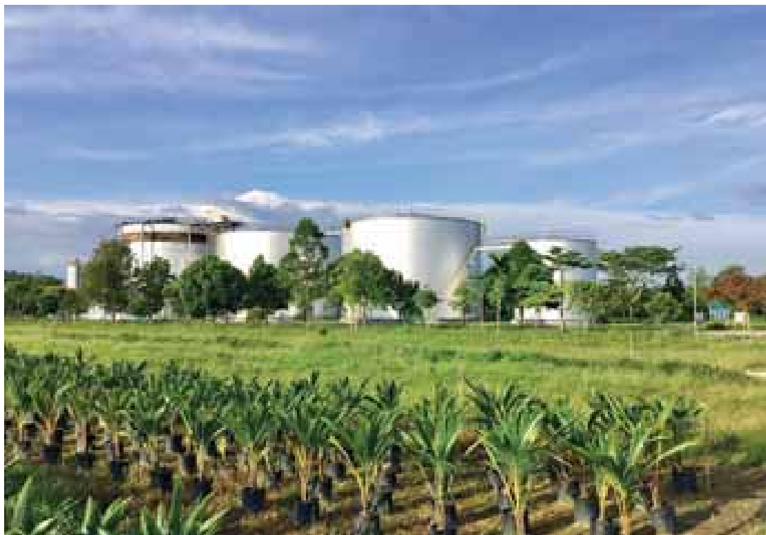
A Biogas Plant at UIE Estate treating the Palm Oil Mill Effluent. In the process of reducing the Biochemical Oxygen Demand by 99%, biogas is produced by methane bacteria and subsequently used as a source of green energy.
