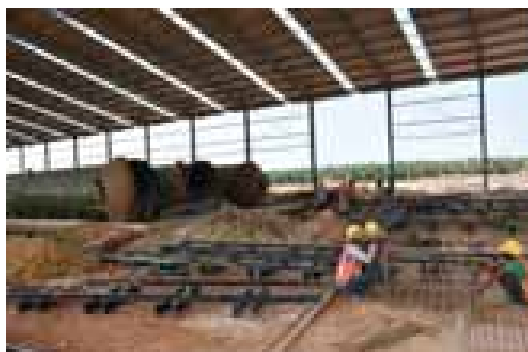
Installation of rail tracks in the marshalling yard.
