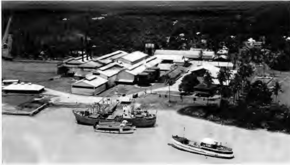
A 12 ton per hour Palm Oil Mill at Ulu Bernam was commissioned in 1932.
