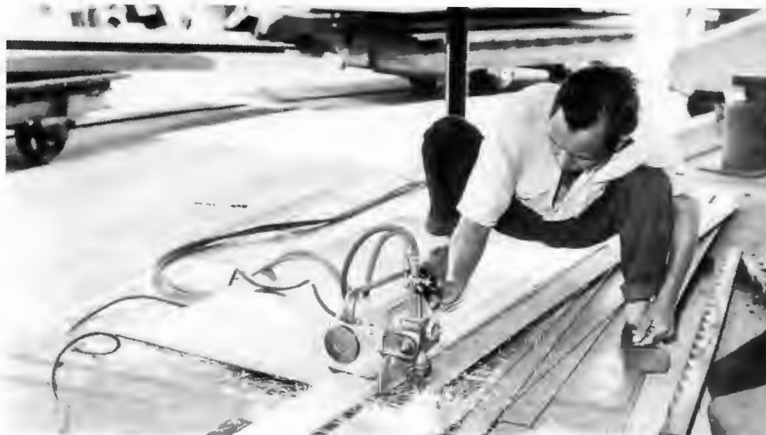
Aligned Oxy cutting of steel plate at Ulu Bernam.
