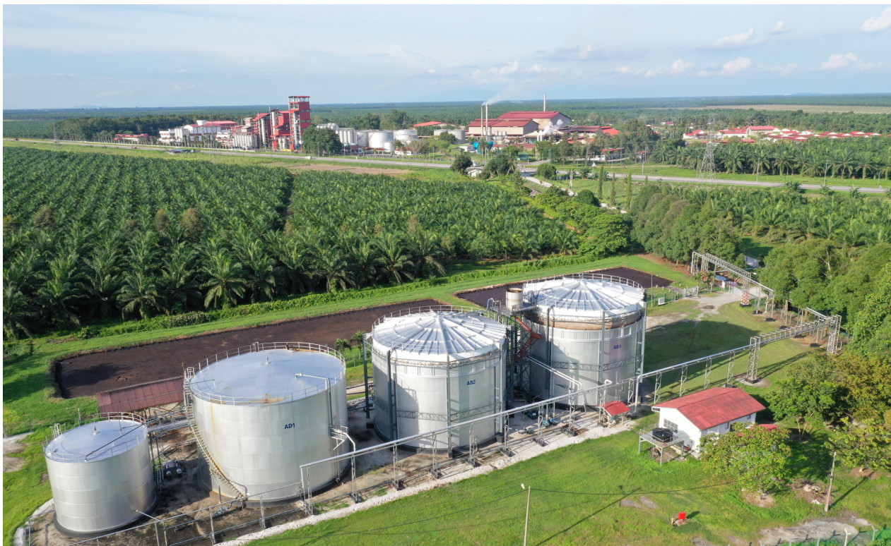
The Jendarata Estate Biogas Plant commissioned in 2006 treating the Palm Oil Mill Effluent. In the process of reducing the Biochemical Oxygen Demand by 99% in Palm Oil mill effluent, biogas is produced by methane bacteria and subsequently used as a source of green energy.
