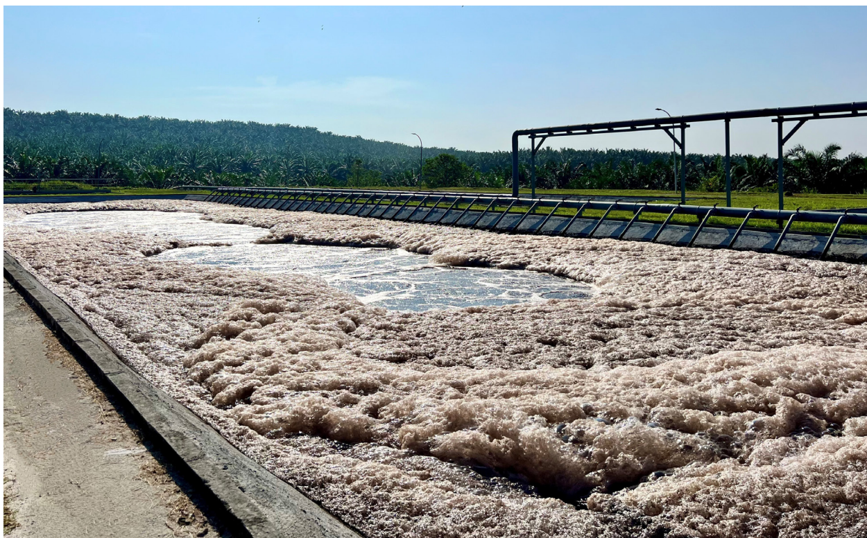
The Palm Oil Mill Effluent Biological Oxygen Demand (BOD) Polishing Plant at the Optimill helps to keep the BOD level below 50ppm after treatment.
